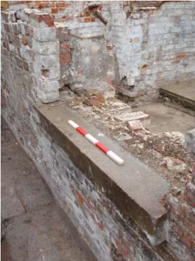
MH17. View of later window cill in Room 8 (looking north-east)
