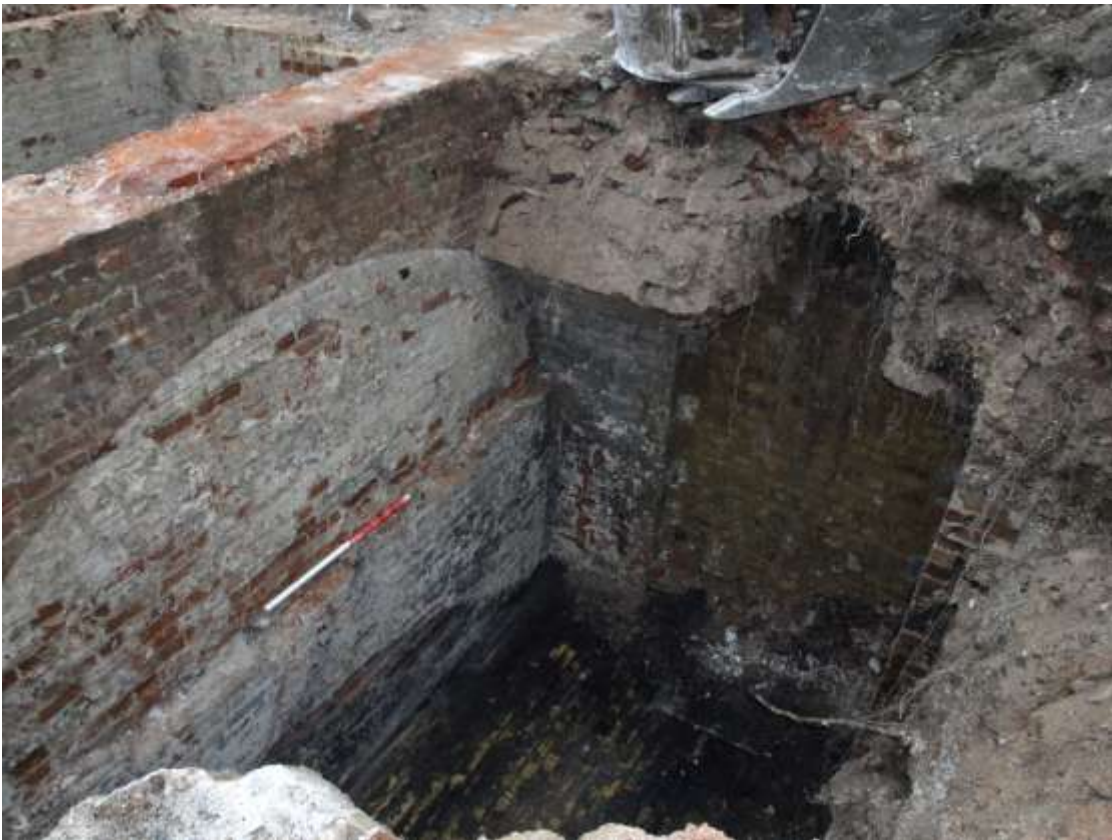
MH1. Corridor 1 (looking north-east. 1m scale)
