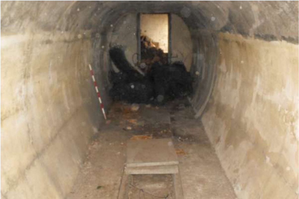
ST16. Area 9. View of air raid shelter (looking north, 1m scale)
