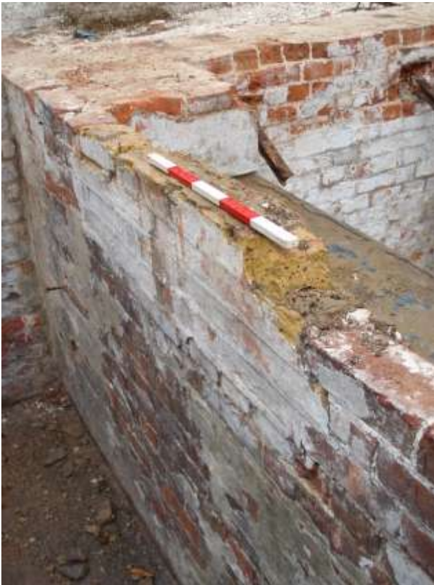
MH16. View of blocked up window in Room 8 (looking north-east)
