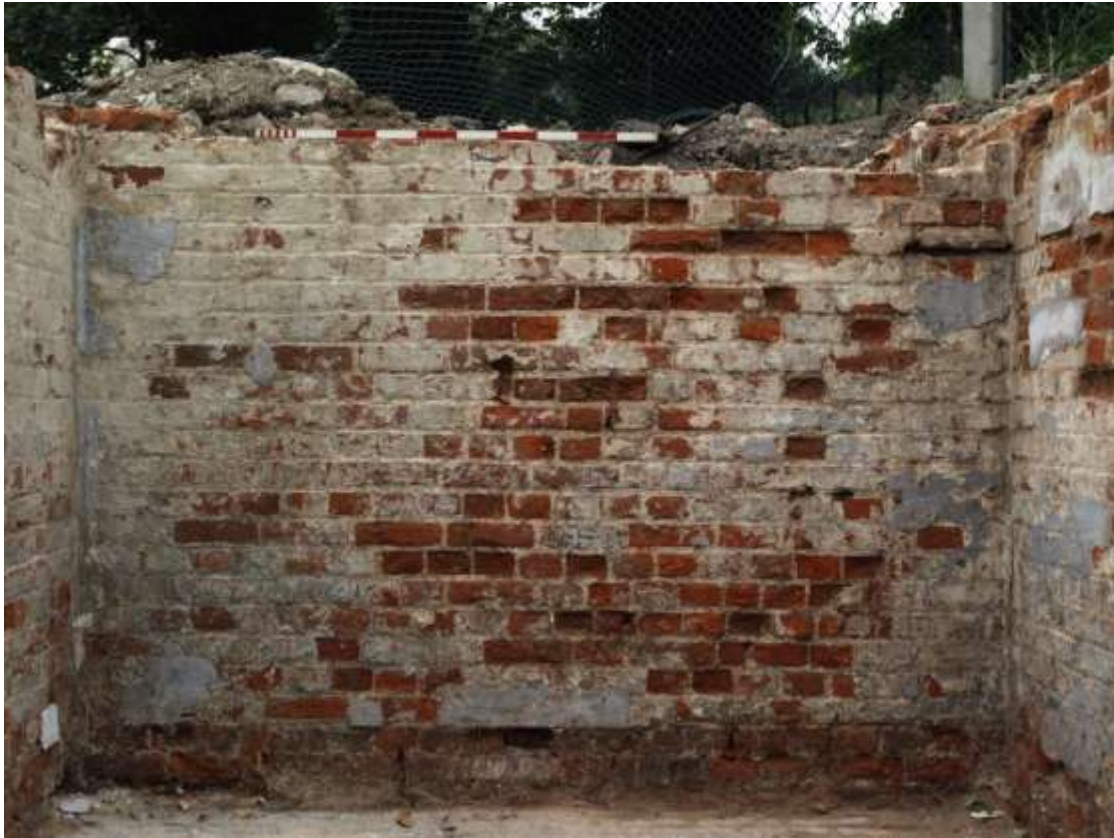
MH5. Room 2: (looking south. 1m scale).
