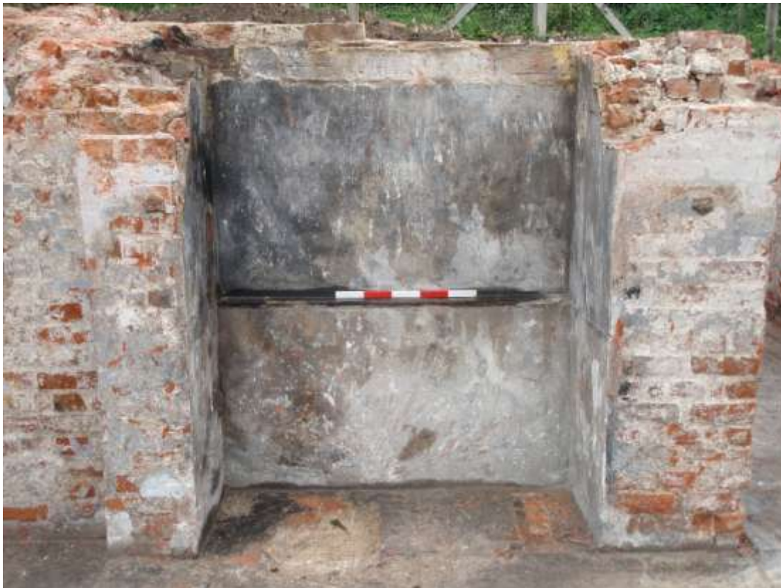
MH8. View of Room 4 (looking south. 50cm scale)
