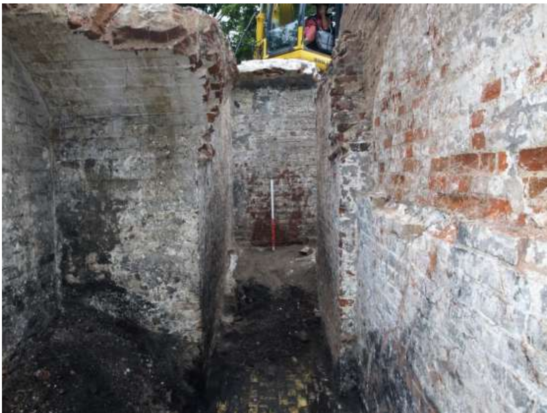
MH2. Corridor 1 (looking west, 1m scale).
