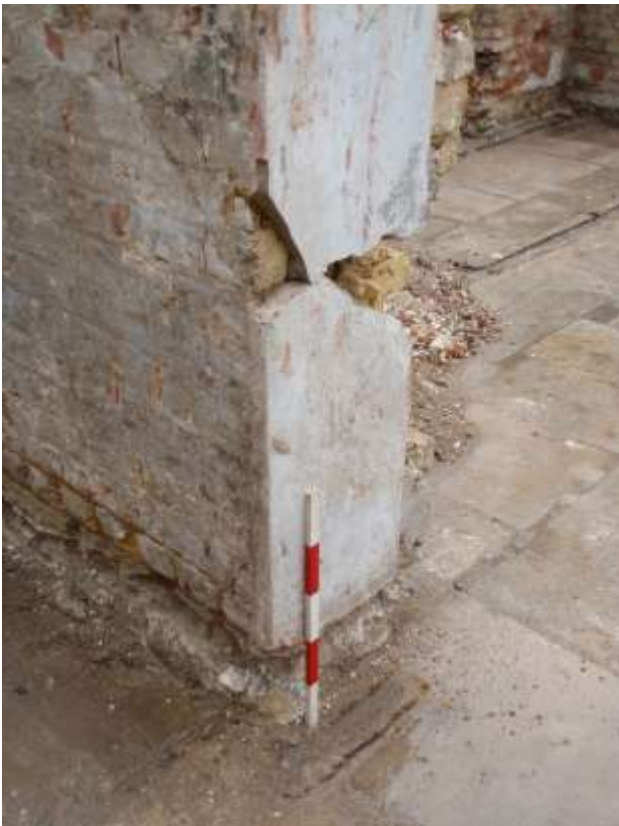
MH18. View of later brick room divide in Room 8 (looking north-east)
