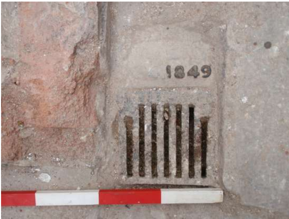
MH22. Detail of drain in Corridor 10. 10cm scale bars
