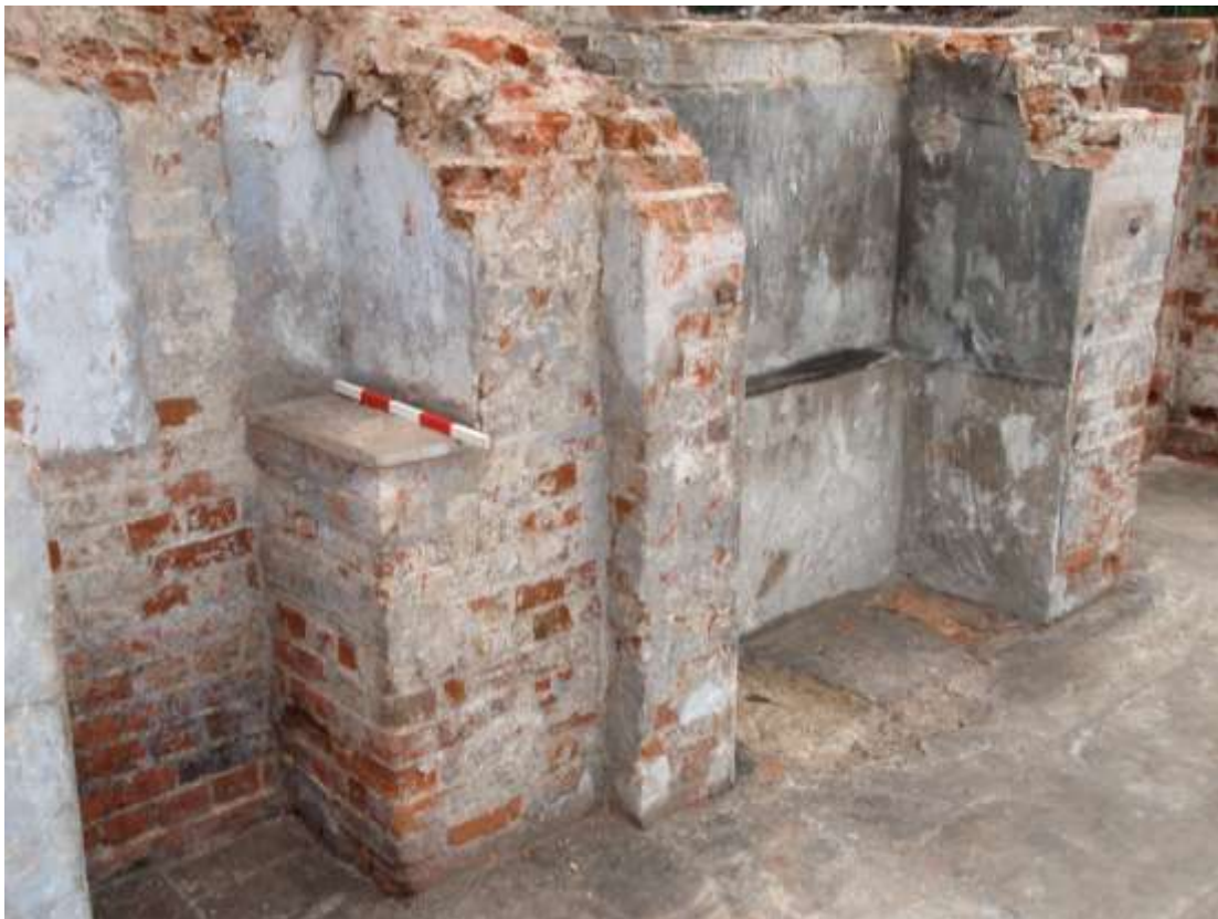
MH10 View of Room 4 (looking south-west. 50cm scale)
