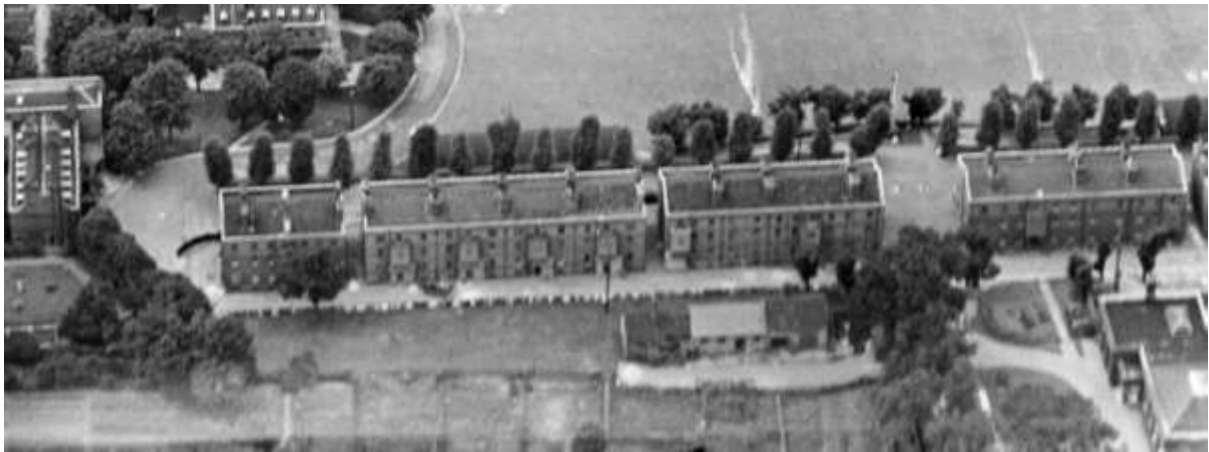
AP 3 taken in 1936 shows the Mess House and adjacent Officers' Quarters. In front of these buildings the Officers' Stables can be seen including the gravel road revealed in the excavations. In front are market garden plots.
