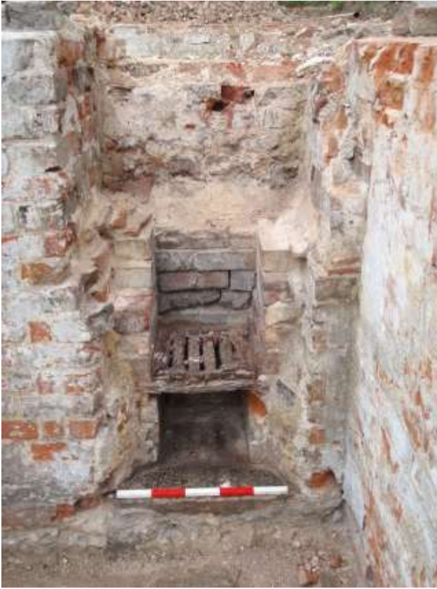
MH15. View of fireplace in Room 8 (looking north)
