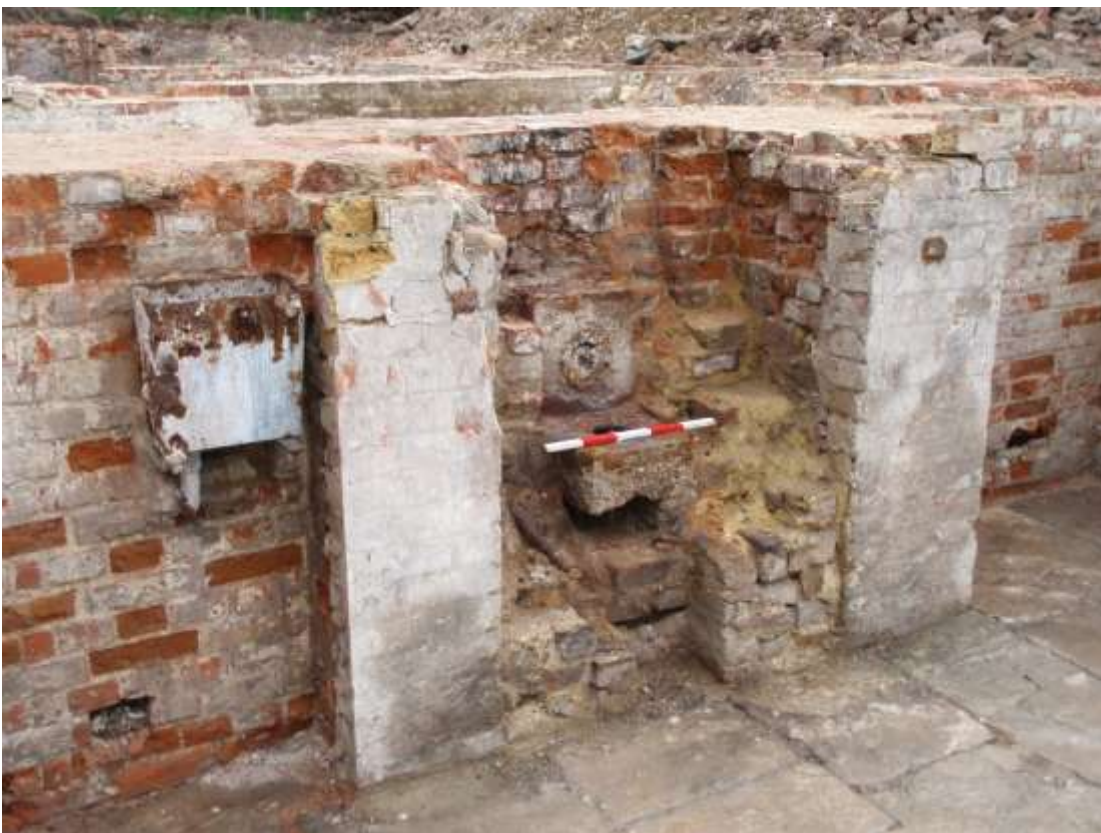
MH25. View of later stove in Room 11 (looking south. 50cm scale)
