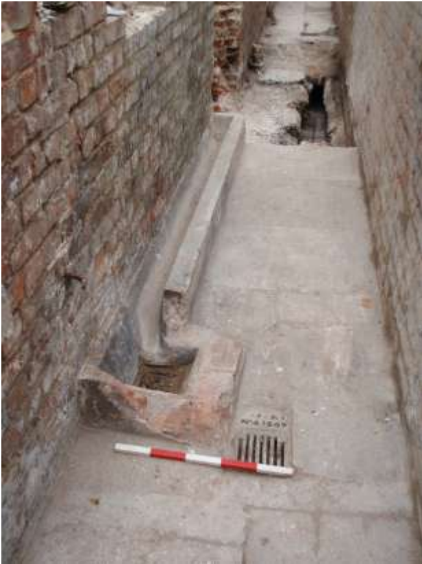
MH20. View of drain detail in Corridor 10. 50cm scale
