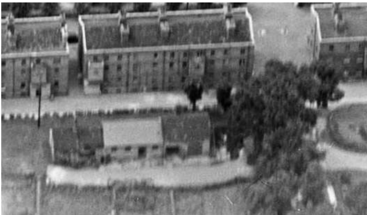
ST2. Detail of the 1936 aerial photograph (looking west)
